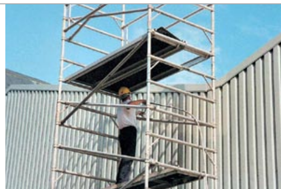
Left: Re-use of pre-finished steel cladding in agricultural application.
