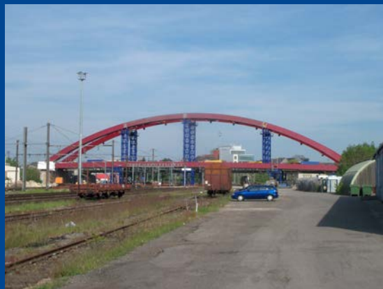
Bowstring bridge - Luxemburg
