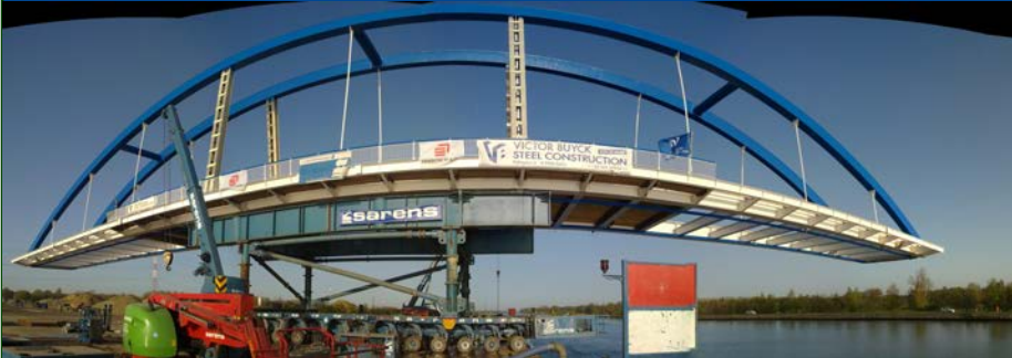
Bowstring bridge over the Albert canal – Grobbendonk (B)
