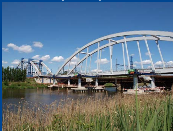
Railway bridges over the river Nete – Duffel (B)
