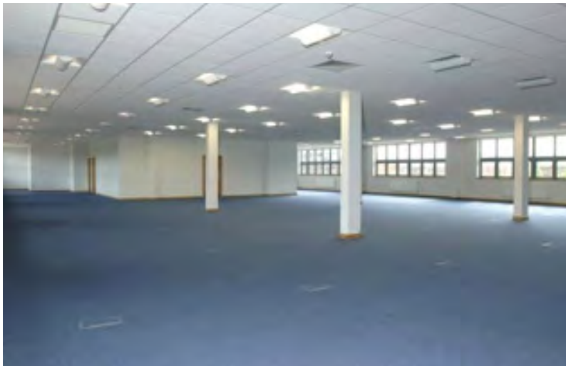
DC3 WAREHOUSE PROLOGIS PARK, STOKE-ON-TRENT OFFICE WING
